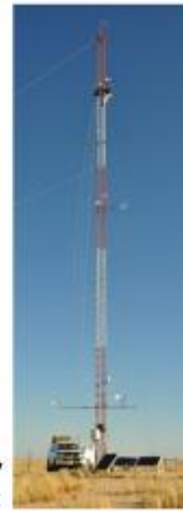
30 m high 'Wind Tower' in the Namib
